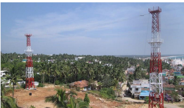
DANPHONE'S NAVTEX SYSTEM IN INDIA
